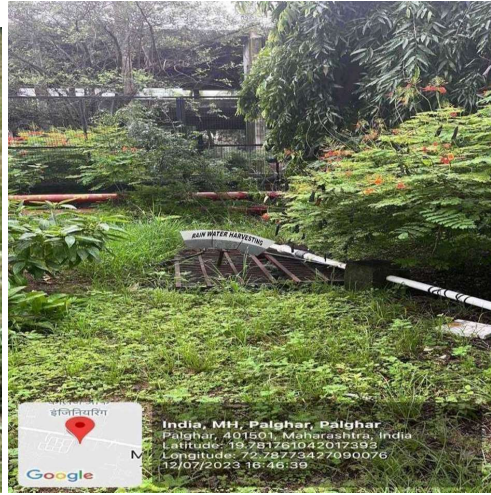
Rain Water Harvesting
